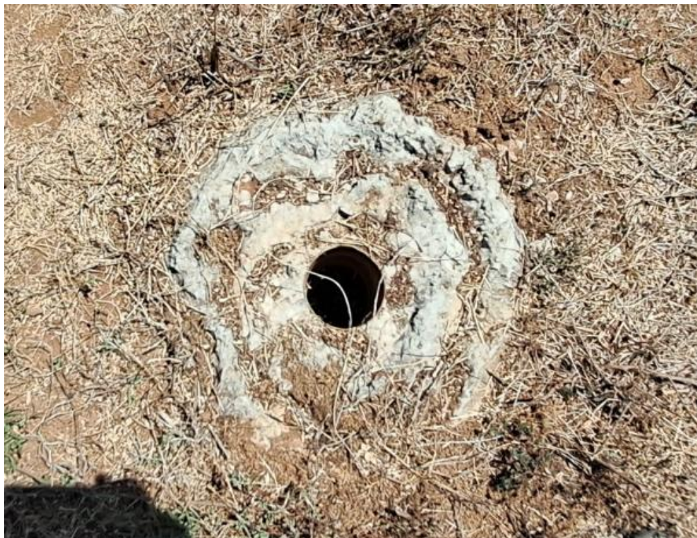
Figure 7.2 Grout holes for grouting through dam body
