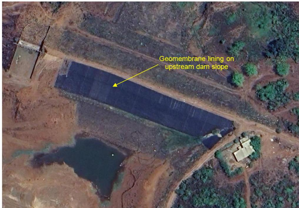
Figure 7.1 Upstream geomembrane lining
