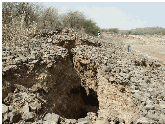
Figure 6.2 Cracking at Shivilakha dam, Gujarat
