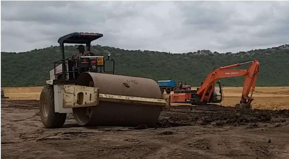
Figure 7.3 Soil Compaction
